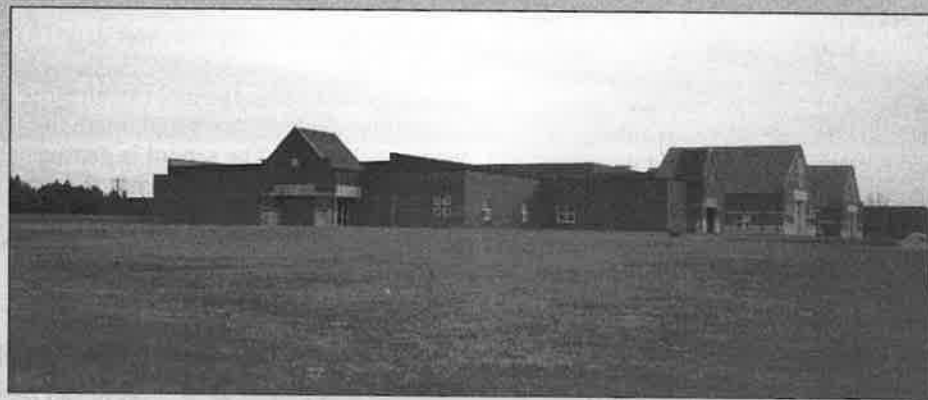
LOOKING FROM THE WEST, the Rock Creek Junior/Senior High School building has some area that it could use for a new expansion. The school board currently has only discussed possibilities and has not yet decided whether an addition will be built or where it would be constructed. PHOTO BY THOMAS McJERNEY
